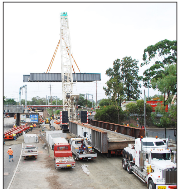
Above - Installation of the new 180 tonne rail bridge beam
