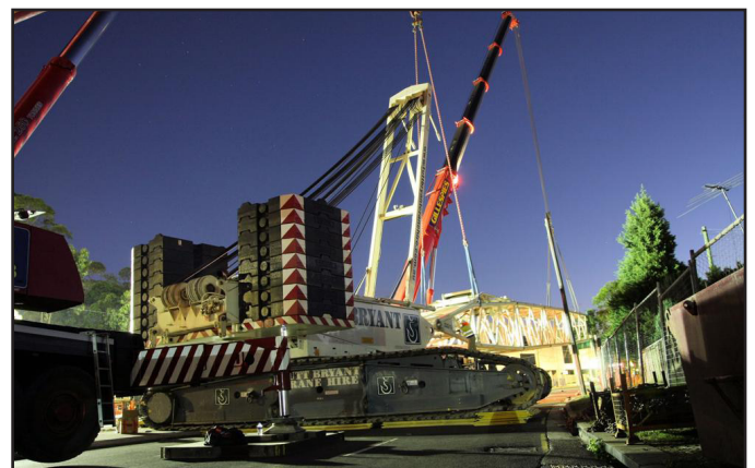
Above - Demag CC2800-1 600 tonne crawler crane
