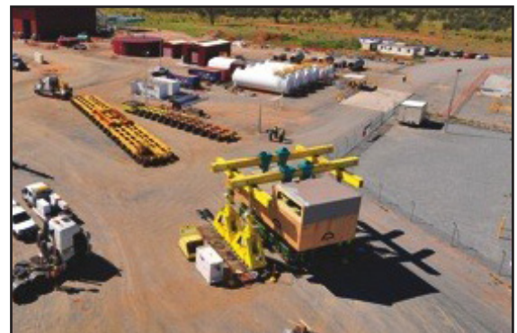
Utilising a modular hydraulic jacking system, Tutt Bryant Heavy Lift & Shift was able to unload and relocate the equipment in one single motion, increasing efficiency
