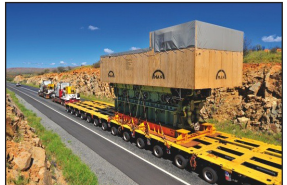
The 230 tonne generator during transportation over the 1,500km journey from Port of Darwin to the Owen Springs site
