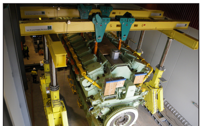
The Hydrospex SBL1100 Modular Hydraulic Jacking System
