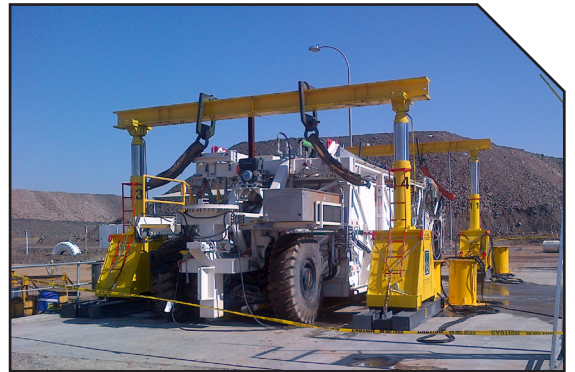
Above - The 4 Point Lift System in operation preparing to lift the undercarriage of the MTM for cleaning.
