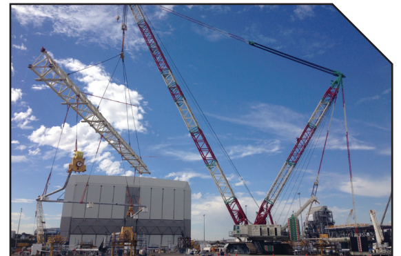
Above - Trial lift of spool data ensuring trouble free subsea installation.
