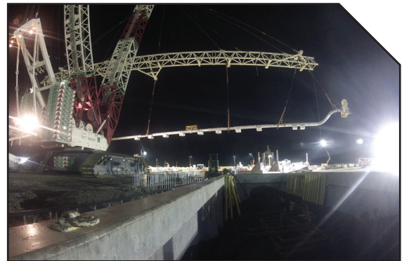
Above - Load out of subsea spool and lifting aid onto barge.
