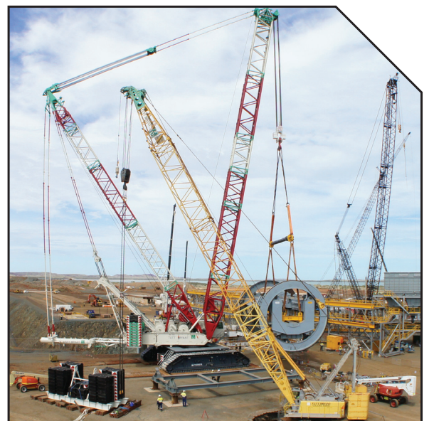
Above - Tutt Bryant's Terex-Demag CC8800-1 Crawler Crane
