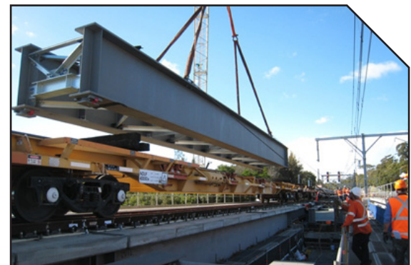
Above - Installation of the new beams
