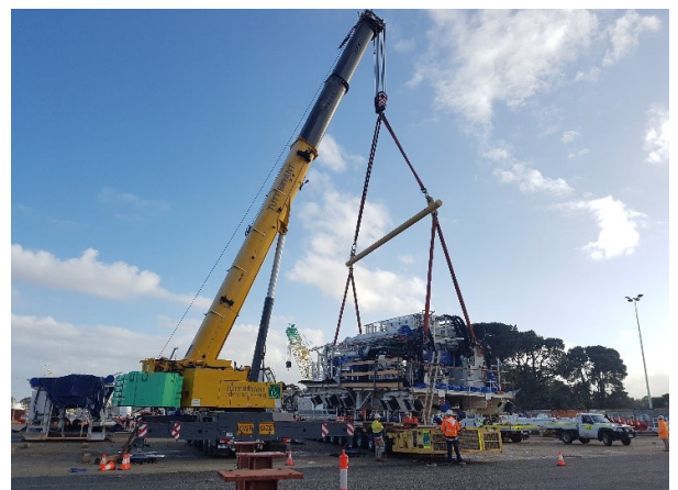
Above: TBHL&S 300t Mobile loading-out 91t Gantry 1 onto the SP trailer
