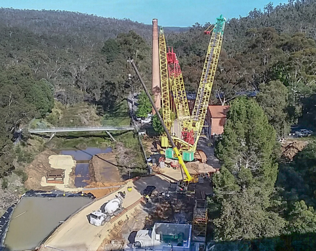
Above: Room is a premium with the M16000 ready to walk down the 10 degree ramp. Top Right: Nicolas SPT used to fit Main Boom Butt and 12 meter boom sections in a very confined space. Bottom Right: Constructing 102 meters of boom down a creek bed.
