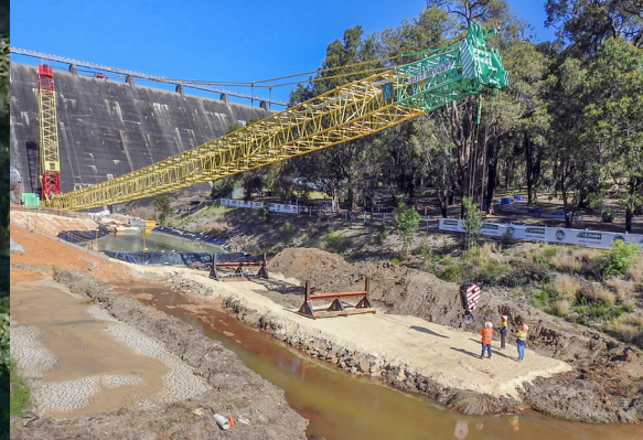
Above: Room is a premium with the M16000 ready to walk down the 10 degree ramp. Top Right: Nicolas SPT used to fit Main Boom Butt and 12 meter boom sections in a very confined space. Bottom Right: Constructing 102 meters of boom down a creek bed.
