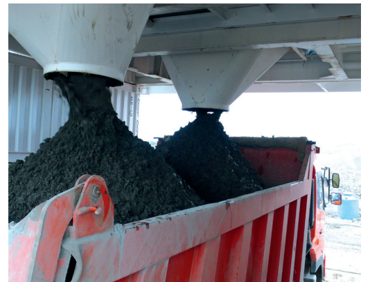
Loading by 2 mixer outlets
